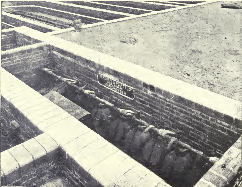
Fig. 41. Distributing Valves.
